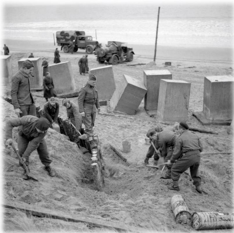
Engineers of the 1st Rifle Brigade (1st Polish Corps) constructing beach defences at Tentsmuir in Scotland. The concrete blocks were used as anti-tank obstacles.
